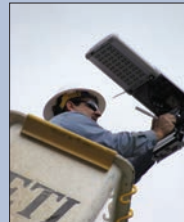
SMPA journeyman lineman Jeff Shea installs an LED street light in Ouray.
