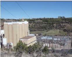
Nucla Power Station.
