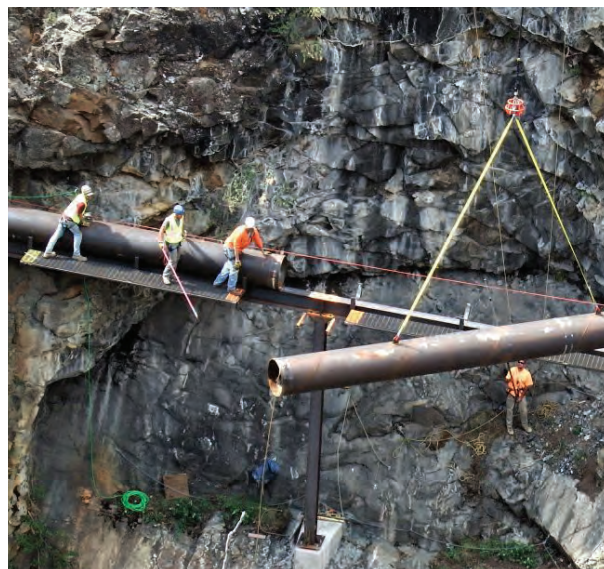
A new penstock is put in place to replace the one taken down by rockfall. Photo Credit: Rick Trujillo
